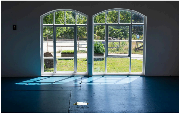
Salettl interior view | © D. Szalai
